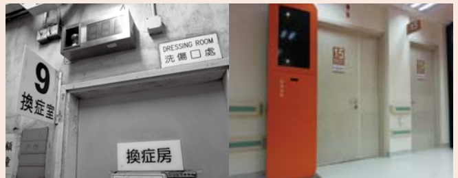
Fig. 4 Treatment rooms of KTJCGOPC and KTCHC
