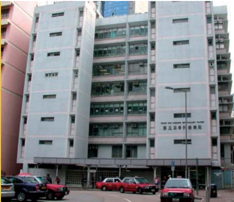
Hong Kong Families Clinic - Tang Chi Ngong Building
